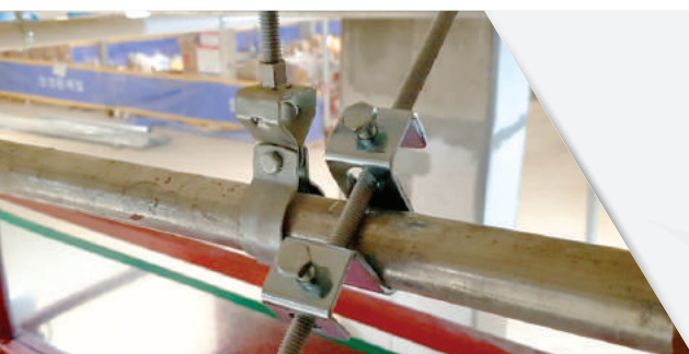
Side Arms Sway Bracing Joint 3/8"
